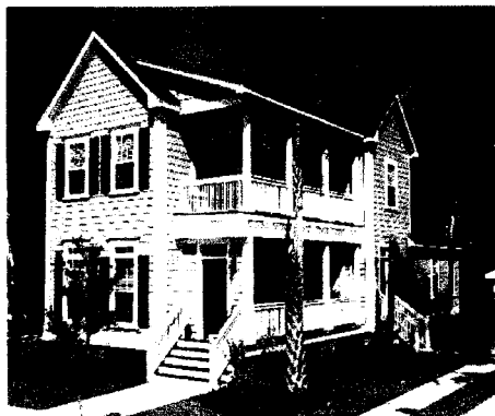
Typical Building Style (Allendale Unit)
