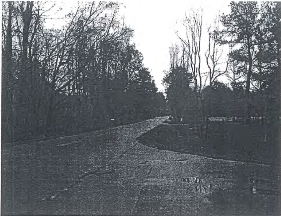
Brownswood Road (Looking South) from Fickling Hill
