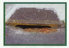
It's the grate or opening next to the curb or sidewalk in to which all the water drains after a storm. In some suburban areas or rural settings, the storm drain system may include open ditches that channel water into waterways, creeks and rivers.
